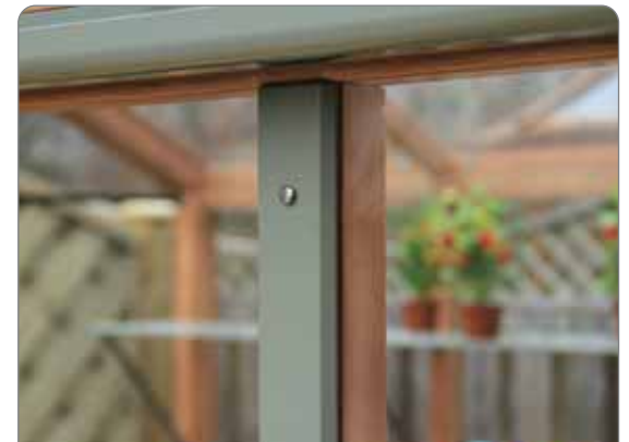
Upgrade to Aluminium Bar Capping
